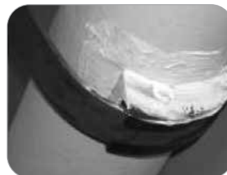
Mastic applied to V-Block saddle at insulation interface. (50°F or greater).
