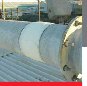
"Rapp-it can be used on all types of pipes including polypipe (PP / HDPE), GRE, ABS, steel, PVC, rubber, concrete, galvanised, ceramic, clay or stainless steel."
