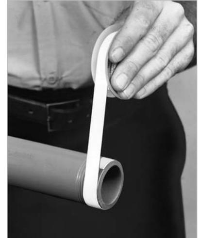
If tape is used, wrap the tape around the entire length of threads beginning with number two thread from the end. The tape should slightly overlap itself going in the same direction as the threads. This will prevent the tape from unraveling when the fitting is tightened on the pipe. Overlapping in the wrong direction and the use of too much tape can affect tolerances between threads. This can generate stress in the wall of female fittings resulting in failure during operations.
