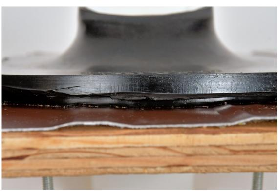
With the Diverting Seal removed you can see how the compression of the Main Seal forms a watertight seal against whatever water gets by the Diverting Seal. On Metal roofs we recommend the Rod Couplings be torqued to 6 ft. lbs. The same principles apply to rubber roofing with compression being key. If there is not a solid substrate between the roof material the Kozy Kollar the Main Seal can not form a watertight seal.
